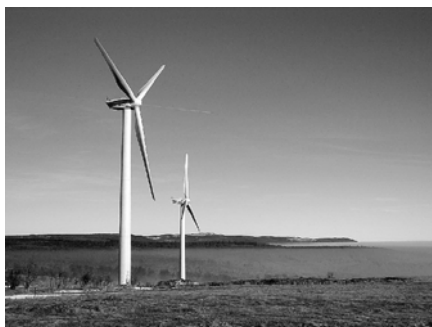
Figure 5 Wind power station in Nova Ves
